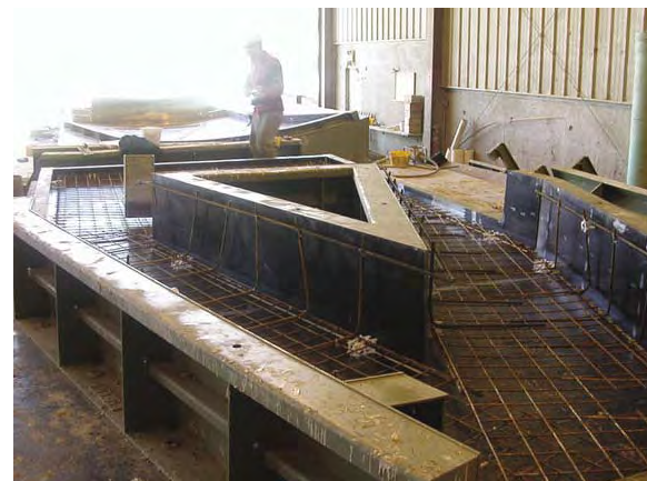
Figure 7: Photo of steel form fabricated by Helser Industries. Photo provided courtesy of High Concrete.
