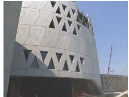
Figure 10: Construction photo of north side of building.
