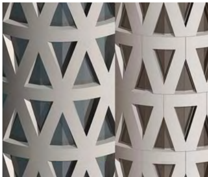
Figure 5: Image of true helical geometry on left and actual modeled solution on right.
