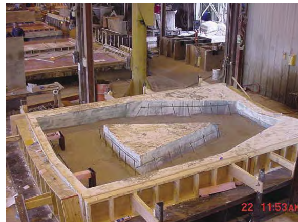
Figure 6: Photo of form made from five-axis milling machine. Photo provided courtesy of High Concrete.
